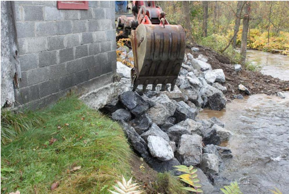
*Stabilizing the barn with rip rap to prevent further loss in the Spring 2014 melt. The project will also entail rootwads and soil lifts upstream of the rip rap to reduce erosion, protect property and enhance habitat.*
