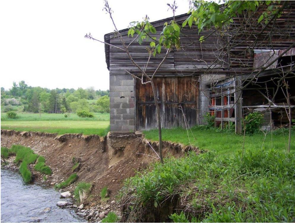
*A streambank on the Mad River in Camden eroding the foundation of a barn.*
